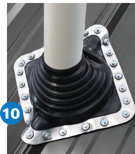
Inspect the installation
