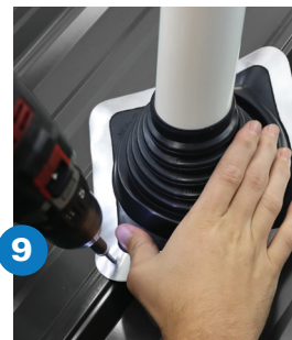
Secure flashing with screws
