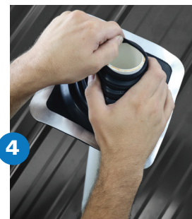
Place the flashing over pipe
