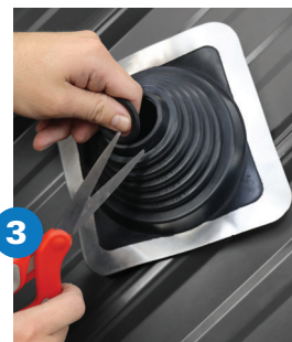
Cut the flashing
