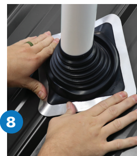
Press flashing onto sealant
