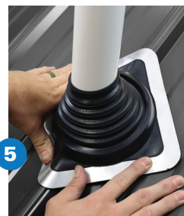
Form the flashing
