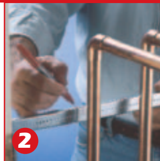
2 Position bracket and mark pipe locations
