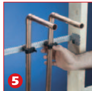
5 Secure the pipe by attaching TPC retainer
