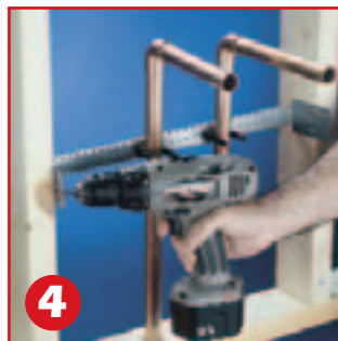
4 Install the TSGB to wall studs
