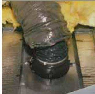
Model DCF The DCF will increase strength and performance for lay in type ceiling applications by transferring weight onto the T-bars. This prevents tiles from sagging over time.
