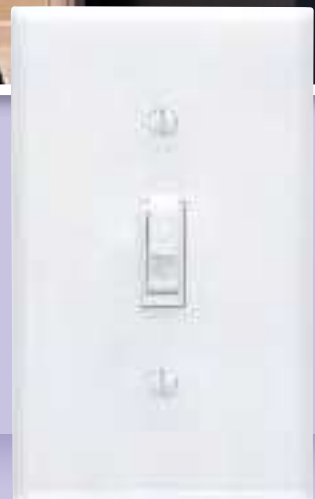
Existing toggle switch
