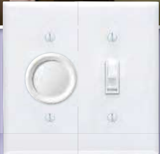
Existing dimmer and toggle switch
