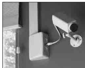
2400 Series Raceway shown with our new 2444D-2N Divided Device Box in a typical classroom application.
