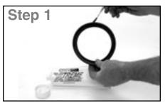
Check & lubricate gasket Check gasket to be sure it is compatible for the intended service. Apply a thin coating of Gruvlok lubricant to outside and sealing lips of the gasket. Be careful that foreign particles do not adhere to lubricated surfaces.
