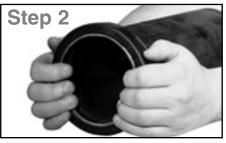
**Gasket Installation** Slip the gasket over the pipe end making sure the gasket lip does not overhang the pipe end.
