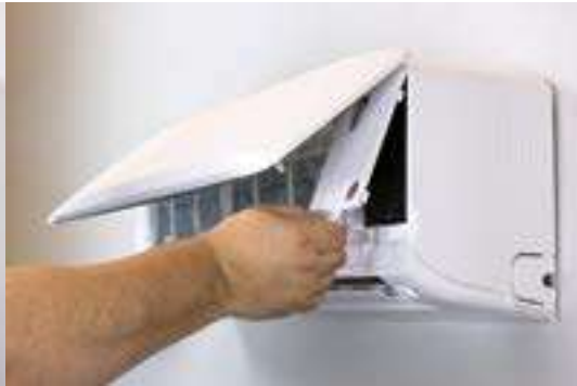
Remove electrical access panels (2)
