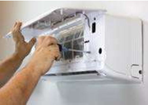
Back out electrical panel screws
