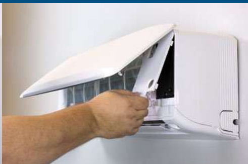
Remove electrical access panels (2)
