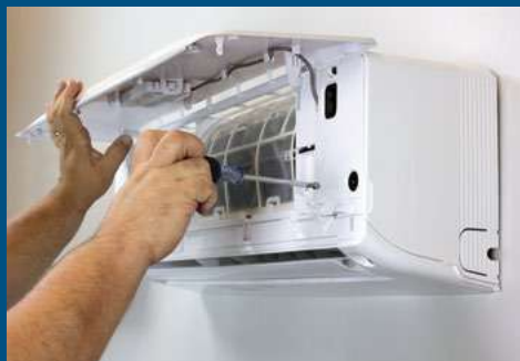
Back out electrical panel screws
