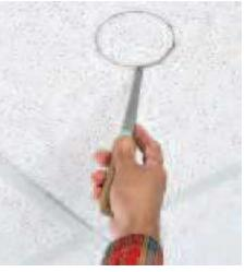
1 Cut a 4-1/16" diameter hole in the center of a 24" ceiling tile.
