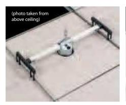
2 Place box over hole. Snap plastic ends of support bar over the ceiling grid (tees).
