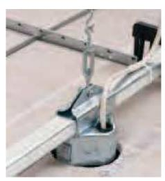
Cable pulled thr ough installed NM cable connector.
