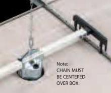
3 Use the "S" hooks provided to attach chain to turnbuckle, and chain to the overhead support. Use turnbuckle to apply tension to the chain, so it supports the weight of fan.
