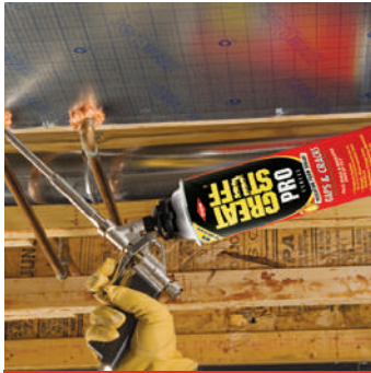
Gas line penetrations
