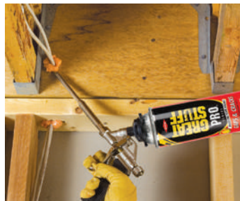
Electrical wire penetrations
