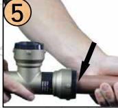
Connection is complete when pipe is fully inserted with depth insertion marked on pipe is still visible at the head of the fitting.
