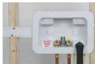
Right drain, box mounted on right stud
