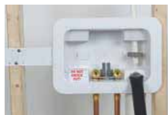
Right drain, box mounted on right stud with secondary drain line
