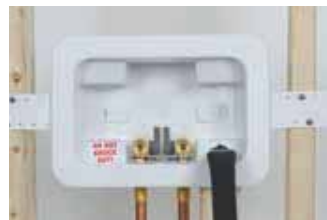
Right drain, box mounted center
