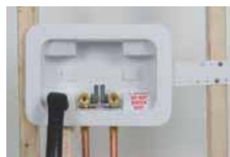
Left drain, box mounted on left stud
