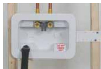
Left drain, box mounted on left stud with valve on top
